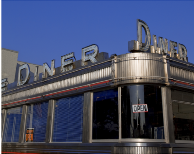
Two signs projecting above roof is not allowed. (Otherwise acceptable design.)
